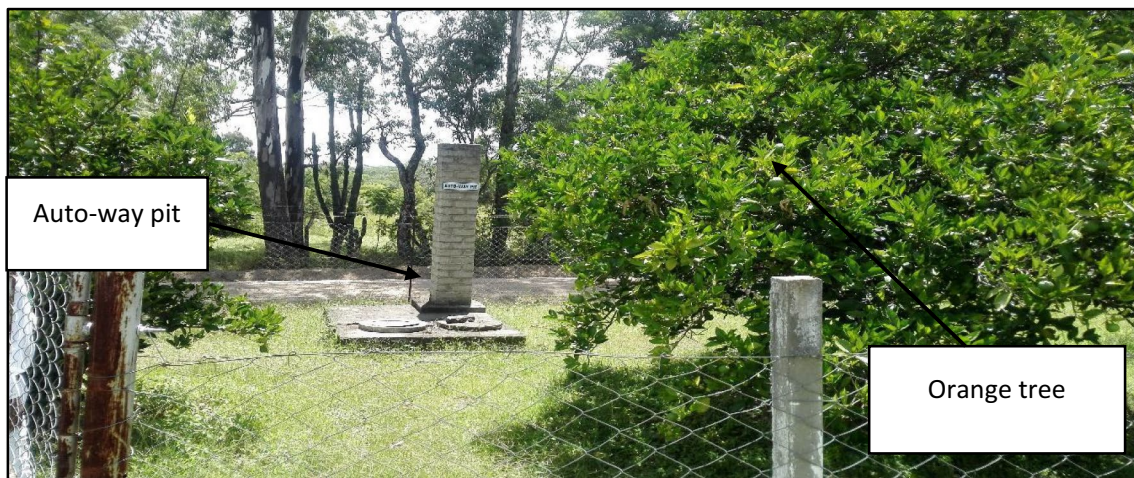
Fig. 18 Autoway pit (located in a minor orchard) used to dispose pathological waste at Holy Cross hospital Source: Field data (2023)
